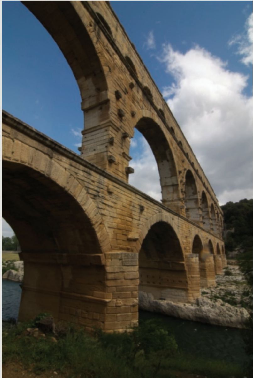
Pont-du-Gard (looking northeast), Nîmes, France, ca. 16 BCE.
